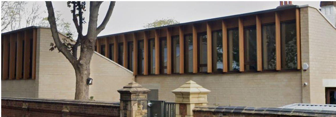
Figure 3: Completed new Sands End Arts and Community Centre
